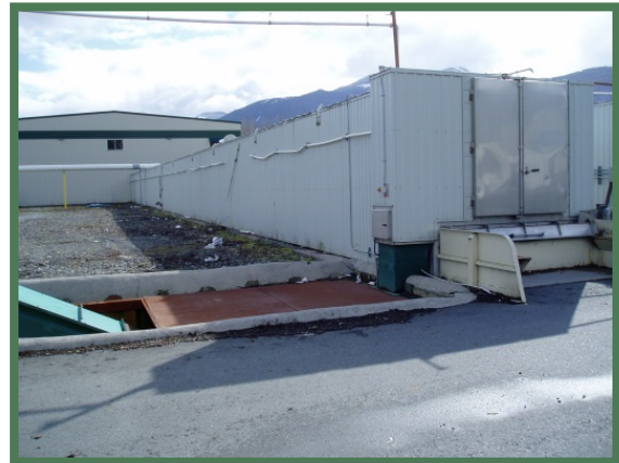
Figure 6: Wright Compost System (agitated container)
