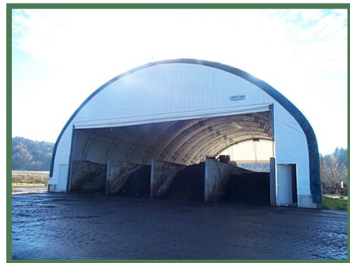
Figure 7: Channel Compost System
